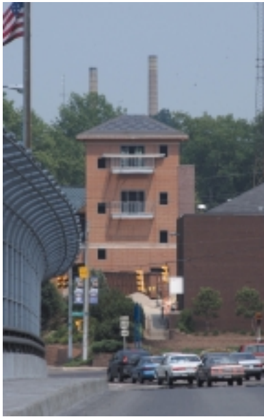
Hose Tower under construction from highway
